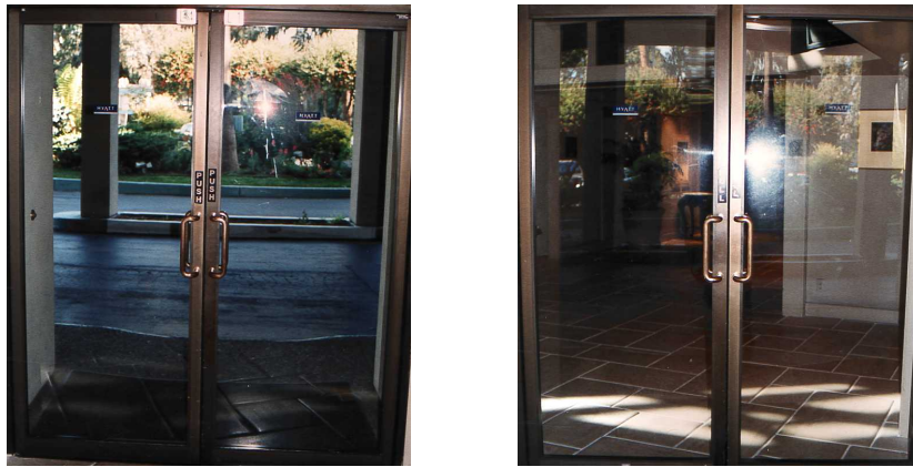
Figure 2.19: An example of ambiguous affordances in door design. The vertical handles mounted on both sides of the door suggest grasping and pulling. Unfortunately, from one side, the door has to be pushed! Note the signs above the handles.
